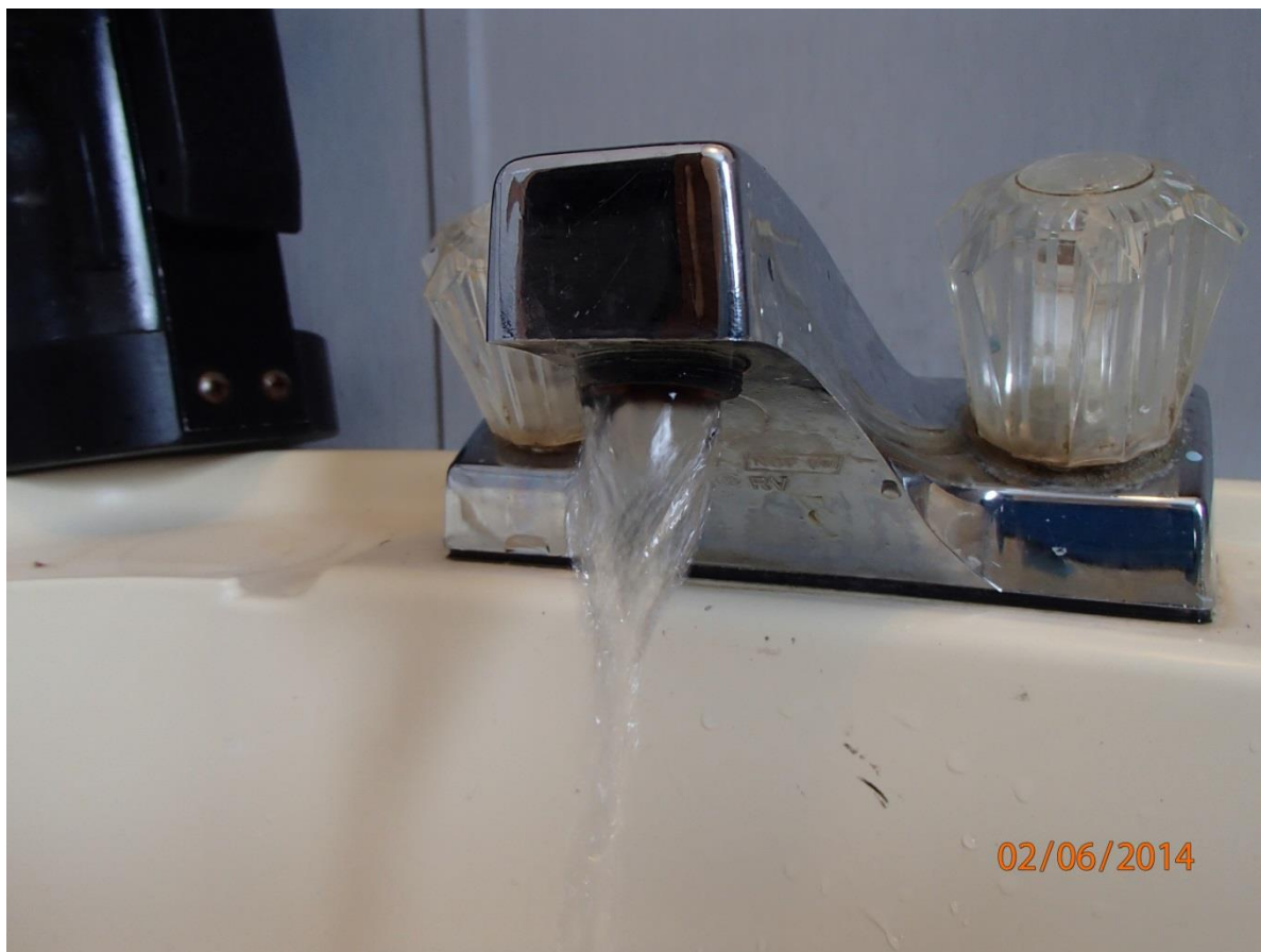
Photograph 1: Up close view of the kitchen faucet with the aerator removed that was used for sampling the spring water for William and Edna Miller's property, parcel # 220000791000, at 20410 Cadiz Road, Freeport, Ohio 43973.
