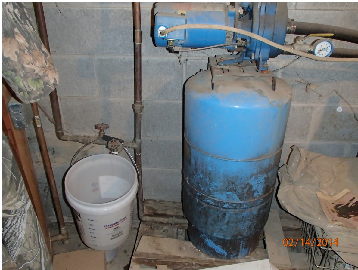
Photograph 1: Up close view of the spigot used for sampling and the pressure tank located directly beside it in the basement of Mary and David Cooper's residence on parcel # 220000047000, at 20411 Cadiz Road, Freeport, Ohio 43973.
